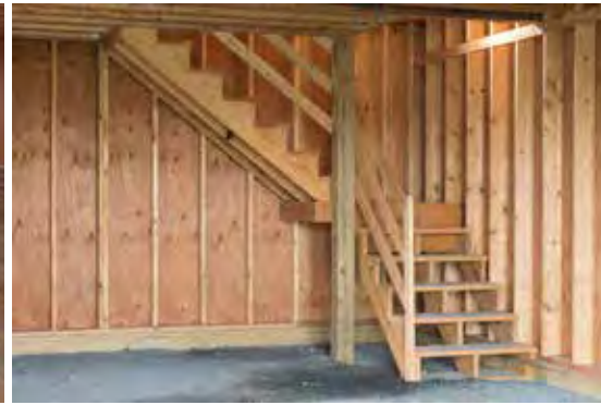
STEPS WITH LANDING AND HANDRAIL
